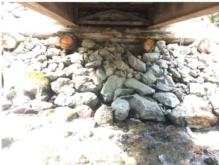
Left Bank Abutment when facing downstream
