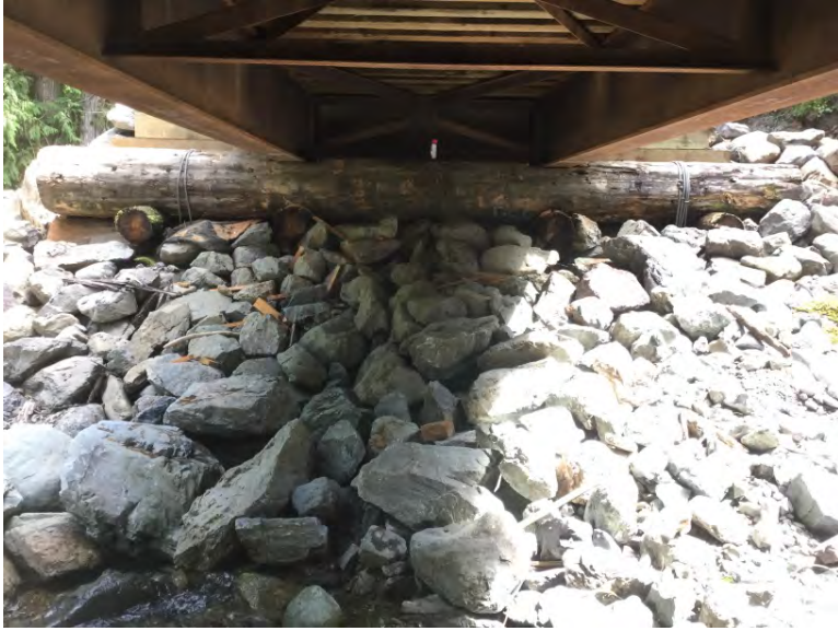
Right Bank Abutment when facing downstream
